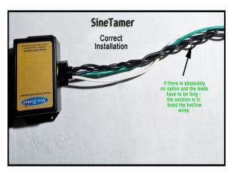
Before energizing, measure the voltage <u>again</u> to insure it is within the levels in the table above. Immediate failure of the surge suppressor will occur if installed on voltages higher than these.
