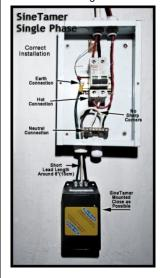
Non-lug type models are provided with 18-24 inches of #10 AWG/TEW stranded wire. For best performance, mount the unit so that all wires can be cut and connected in the shortest and most direct path possible. For every inch of conductor added to the installation, you increase the letthrough voltage of the suppressor by about 10 volts for an ANSI/IEEE Category B, 6 kV, 3 kA impulse.
