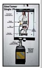
**Note:** If necessary for additional wiring flexibility, the ST-SPTxxx-15 can also be connected in parallel, by connecting either of the two terminal sides available. The exact protocols listed above must be followed. Connection leads must be a short and straight as possible.
